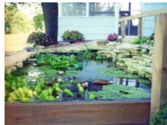
Using strong support posts, one end of his grandparents' pond is constructed with a strong, wooden retaining wall that allows Josh to get up close and personal with the pond.
